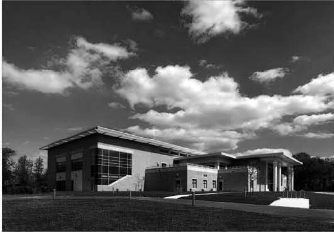
WEST COUNTY LIBRARY ODENTON, MARYLAND
